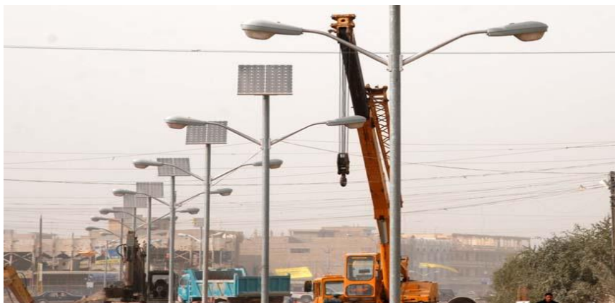
Figure-3. Installation of PV solar streets lighting in Iraq
