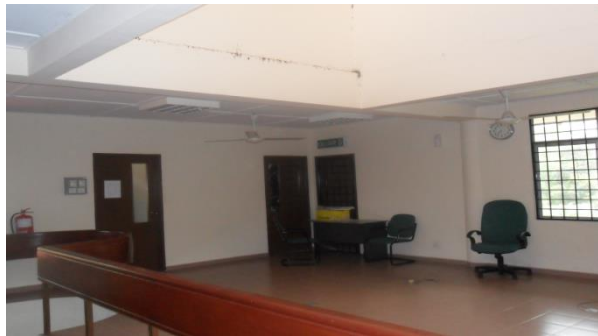
Figure-2. Interior Condition of TSM
