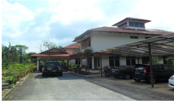
Figure-1. Tapak Semaian Mantin (TSM) office building and its surroundings
