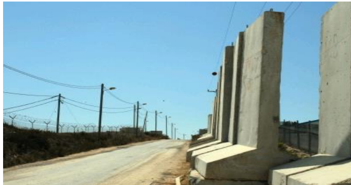
Fig-1. Typical reinforced concrete blast wall [1]
