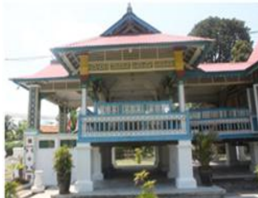
Figure-4. Verandah is enclosed by balustrades and built on stilts to create more airflow to the house.
