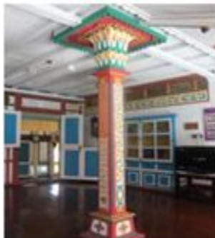
Figure-6. The rumah ibu (main house) is the most important part in the architecture of a traditional house. This is where the ‘main pillar’ or tiang seri is located.
