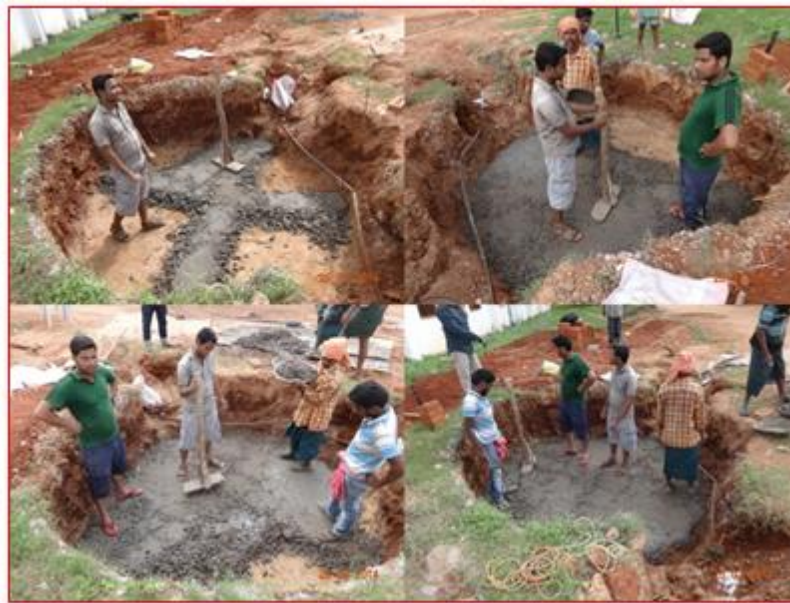
Fig-3. PCC work in progress
