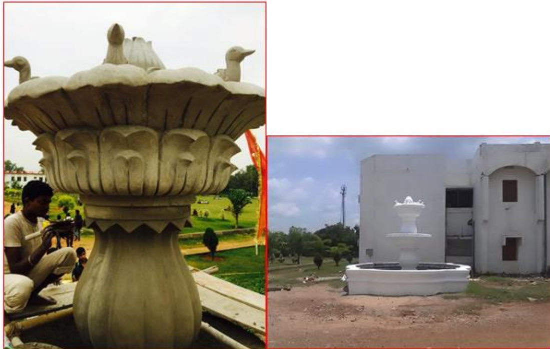
Fig-8. Finishing and ornamental work in progress
