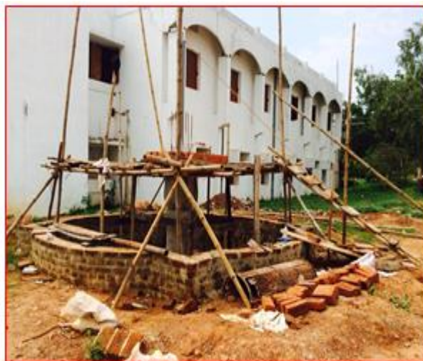
Fig-5. Scaffolding and shuttering Source: Orissa Engineering College Campus
