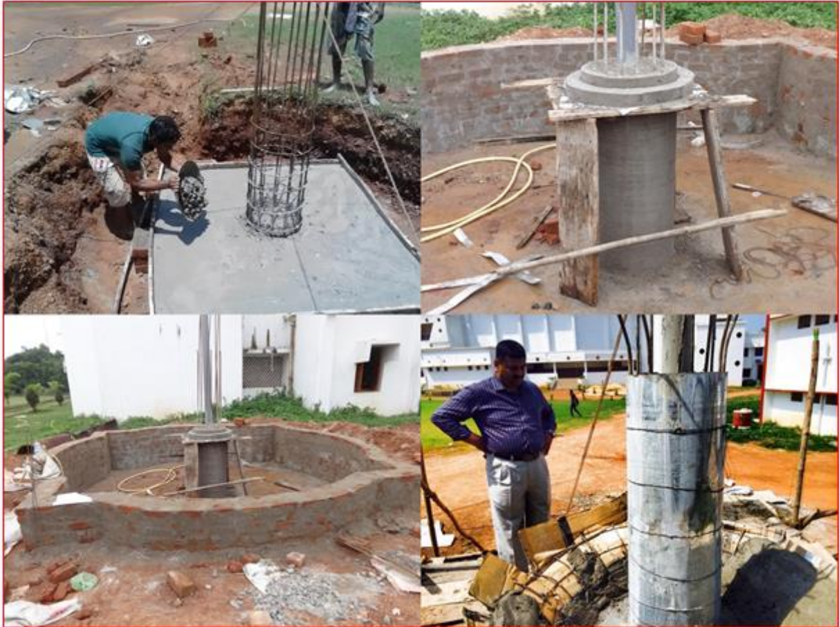
Fig-7. Phase wise proceeding of central column
