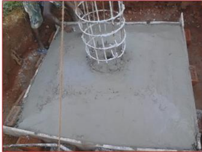
Fig-4. reinforcement and erection of column Source: Orissa Engineering College Campus
