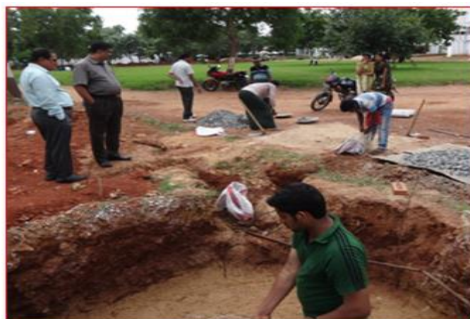
Fig-2. Sand filling and compaction
