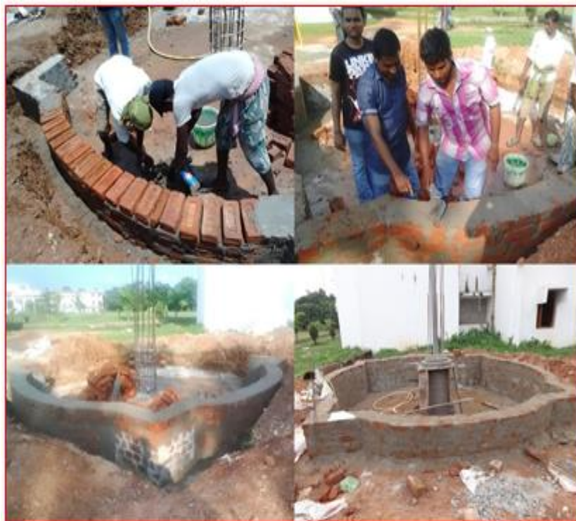
Fig-6. Brick work in full swing
