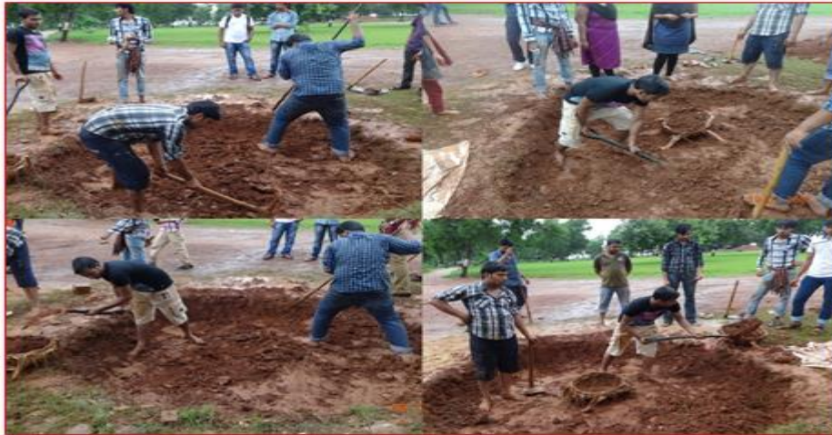
Fig-1. Excavation work in progress for the foundation
