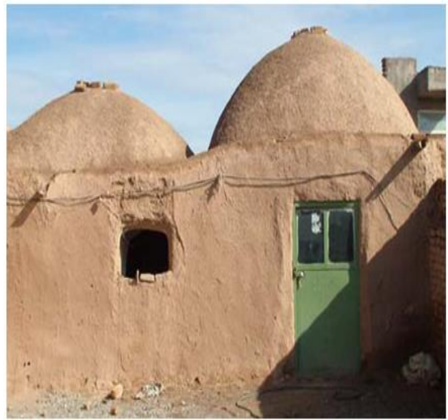
Figure-2. Vernacular domed houses in Iran
