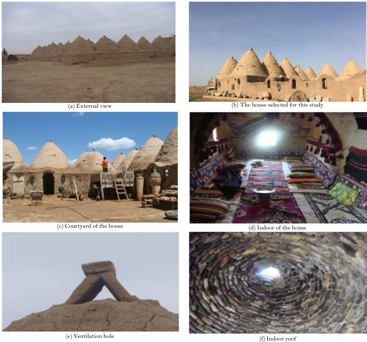
Figure-6. Parts of the Harran vernacular domed houses
