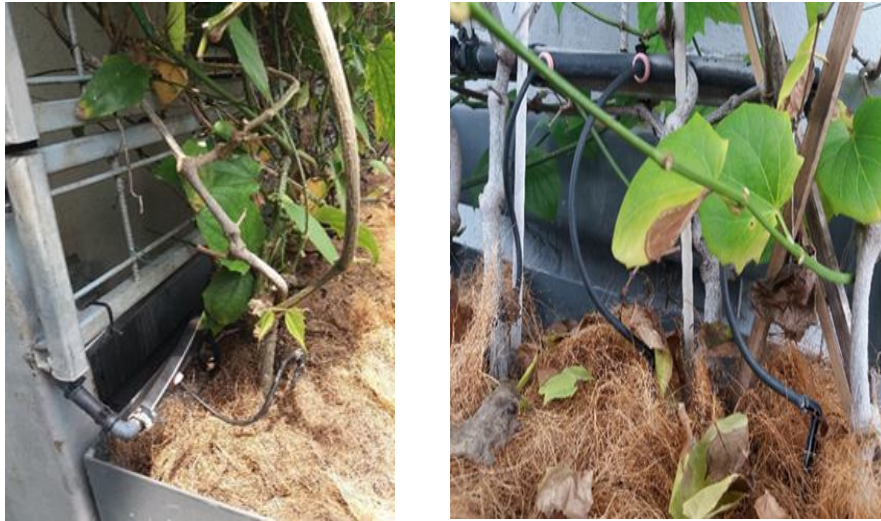
Figure-3. Views of a green wall using a drip irrigation system.
