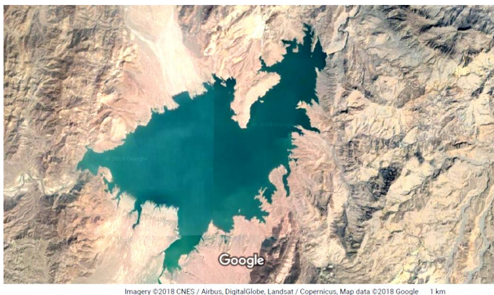
Figure 1: Ariel view of Gomal Zam dam
