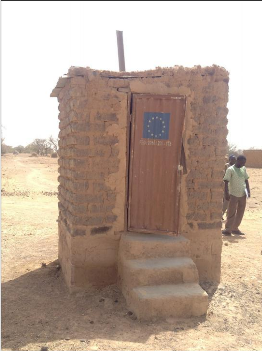
Figure-1. Latrine Ecosan with at the back the sensitization agents and beneficiaries
