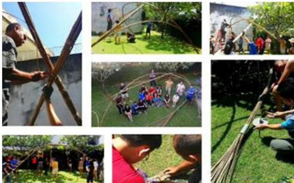
Fig-8. On-site construction of Pavilion NOW 2015 (SGFA, 2015)
